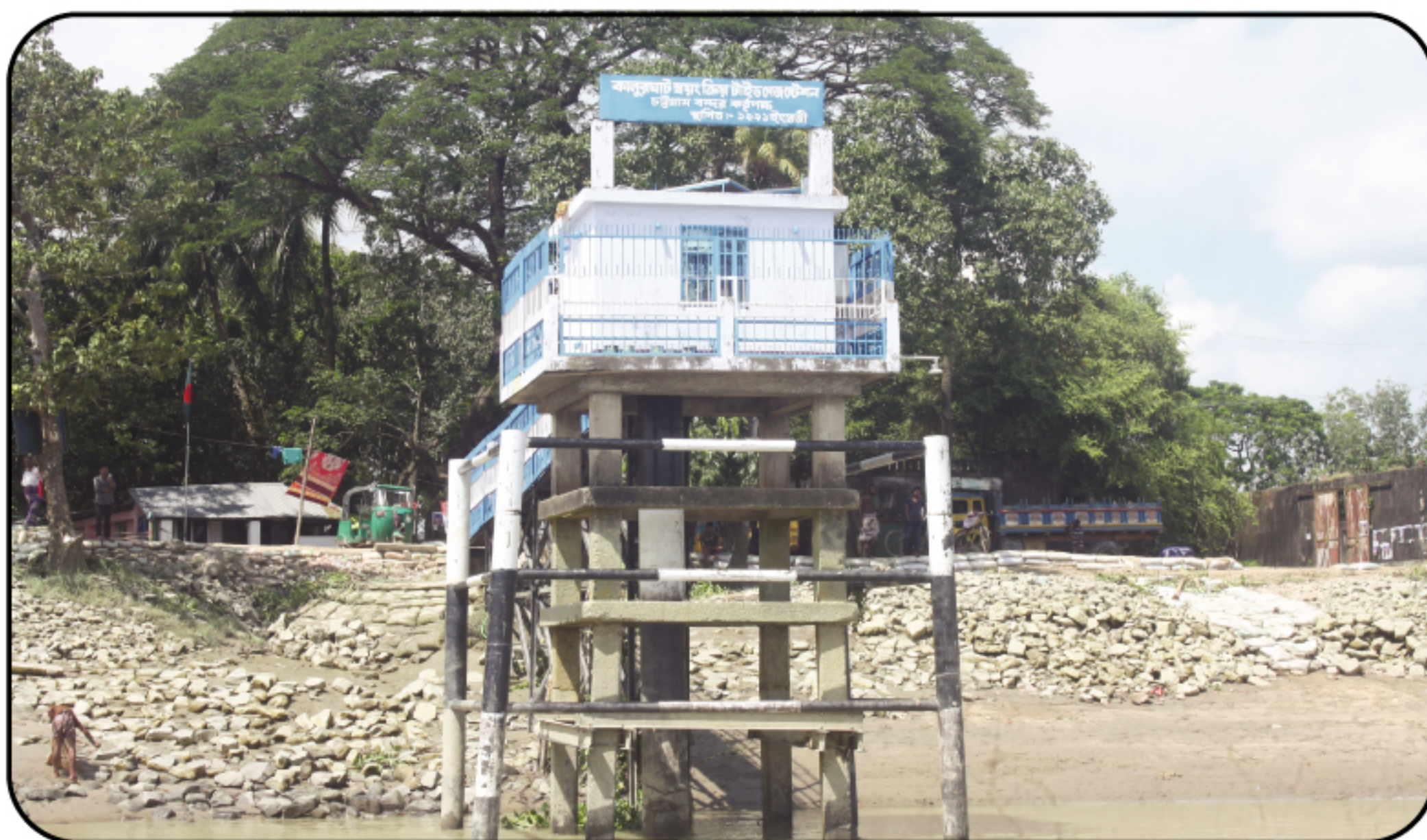
Auto Tide Gauge Station at Kalurghat
