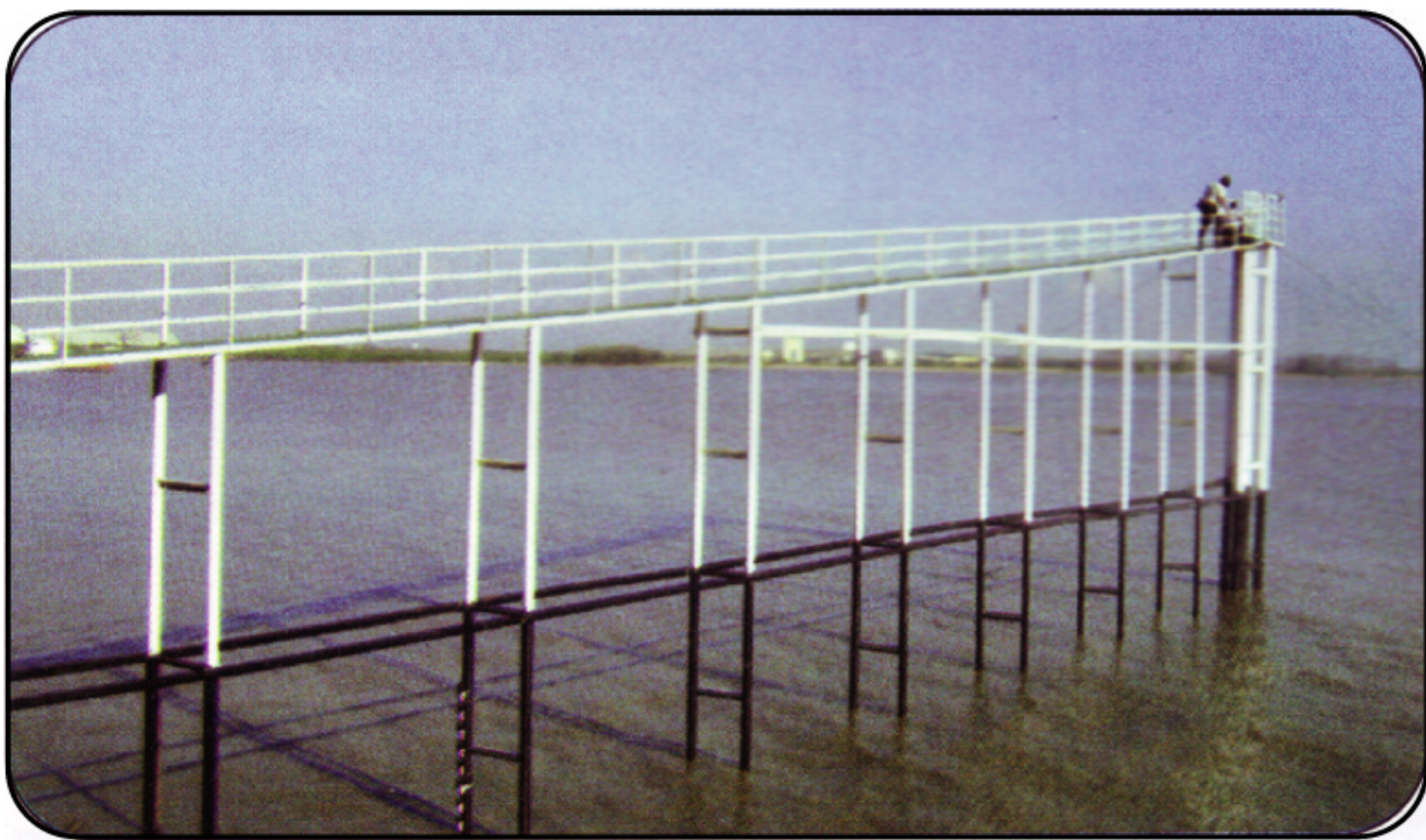
Auto Tide Gauge Station at Khal 18
